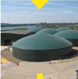
**The liquid food waste is then transferred to large tanks where it is continuously stirred for over 100 days. During this process gasses are released from the liquid including methane and carbon dioxide.**
