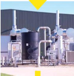
**The methane extracted from the tanks is fed into gas engines to generate renewable electricity and heat.**
