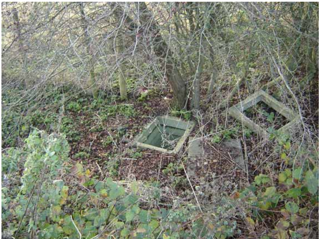
Area 1- Blackditch culvert corner Blackditch Road and B449
