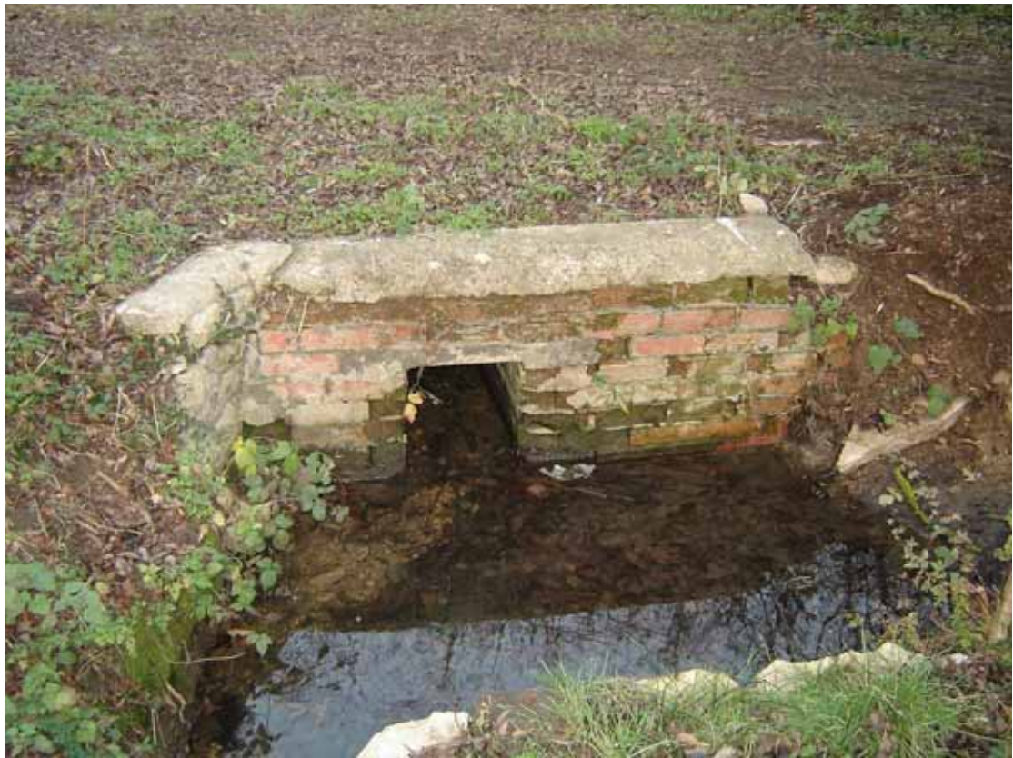
Area 2 - Sutton Pond Pipework Inlet
