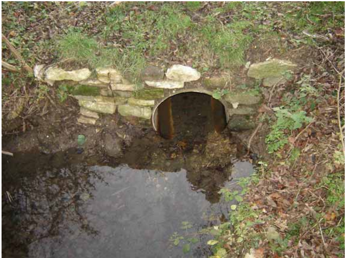
Area 2 - Sutton Pond Pipework Inlet
