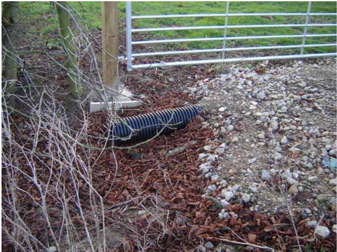
Area 1 - Stanton Harcourt Road field entrance
