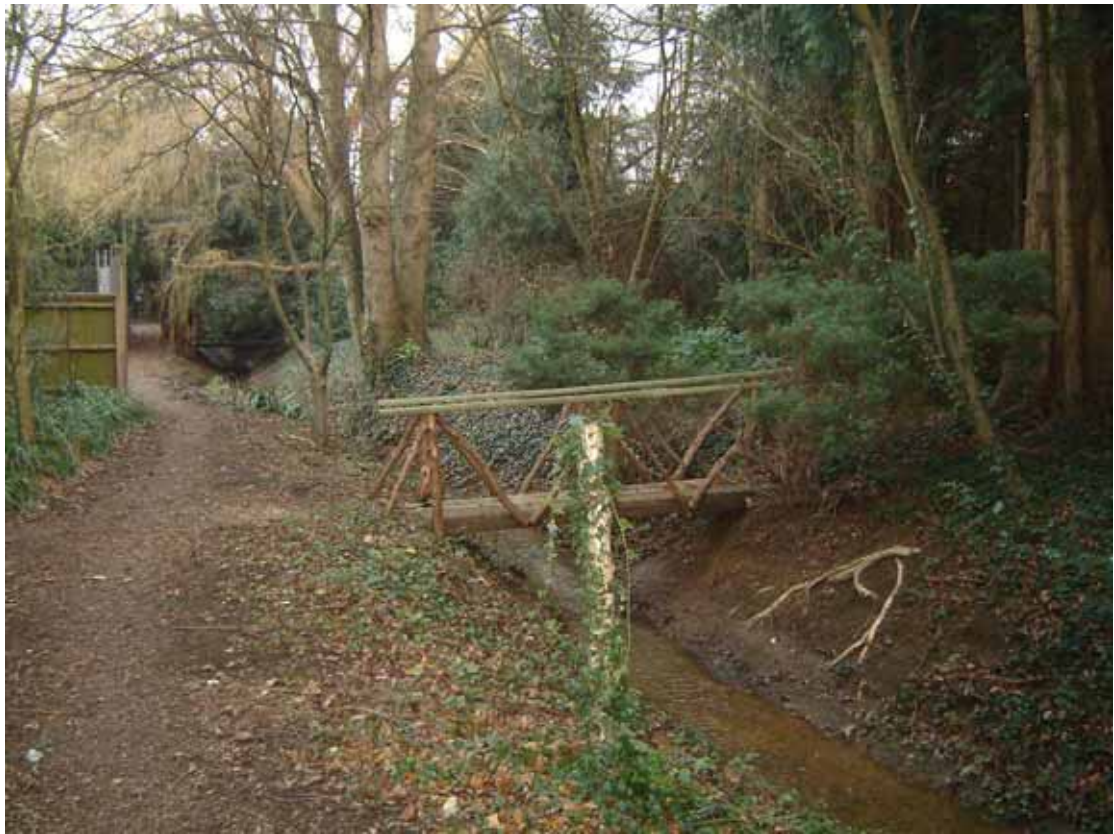
Area 1 - Blackditch open watercourse through Blackditch Farm
