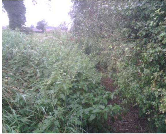
Area I - Perimeter ditch of recreational field. This is on the southern side
