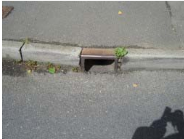
Area 2- Highway Drainage outlet opposite Foxwell Court
