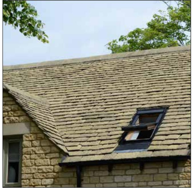
Fig. 7 Artificial stone slate roof with flush roof-light
