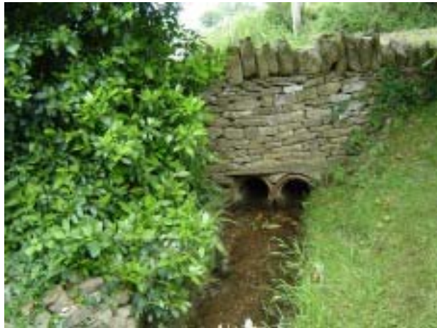
Area 4 - Field wall at Greywalls
