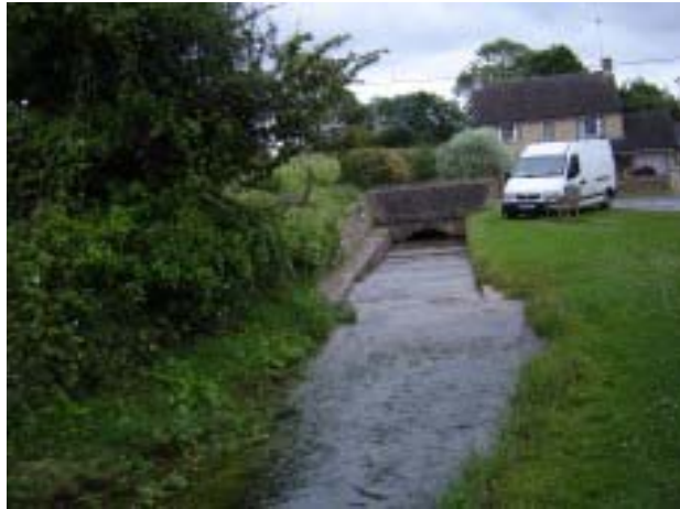
Area 1 - Brook course culvert Brook End
