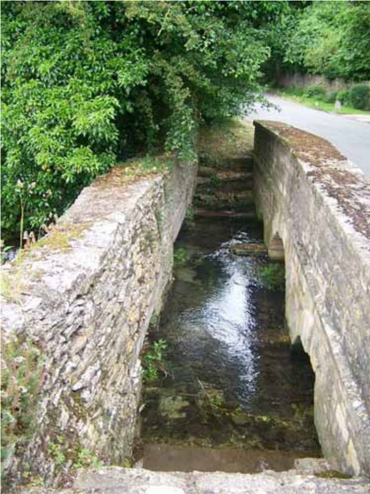
Photograph 7: Bridge Street Bridge upstream face
