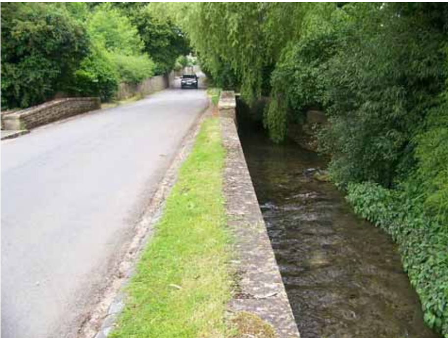
Photograph 8: Bridge Street Bridge showing downstream channel running parallel to road
