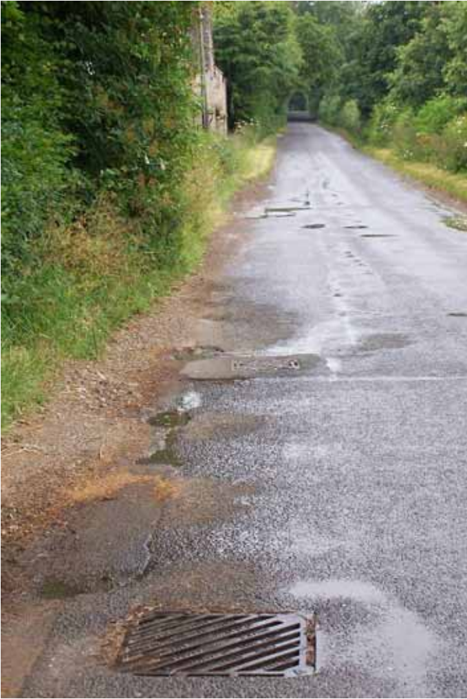
Photograph 25: Drainage along road, looking away from Shilton
