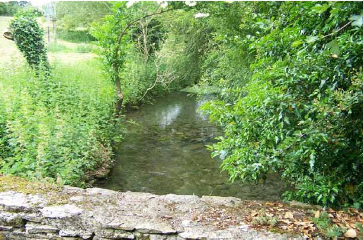
Photograph 6: Bridge Street Bridge, looking upstream of Shill Brook
