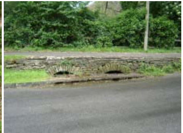
Area 2 - Highway drainage outlet to recreation ground
