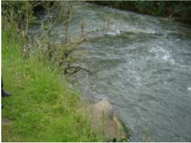
Area 2- Recreation car park drainage outlet
