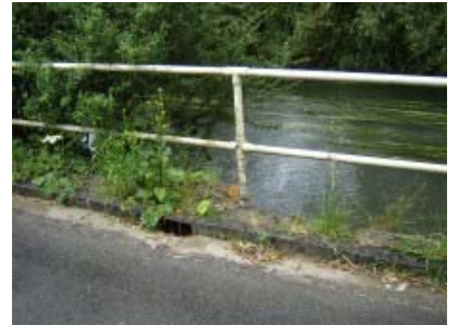
Area 2- Mill stream bridge in High Street
