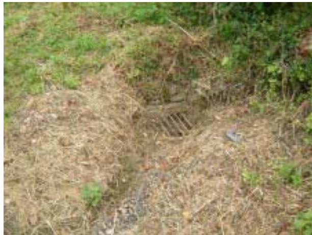
Area 2- Drainage Gully in the High Street
