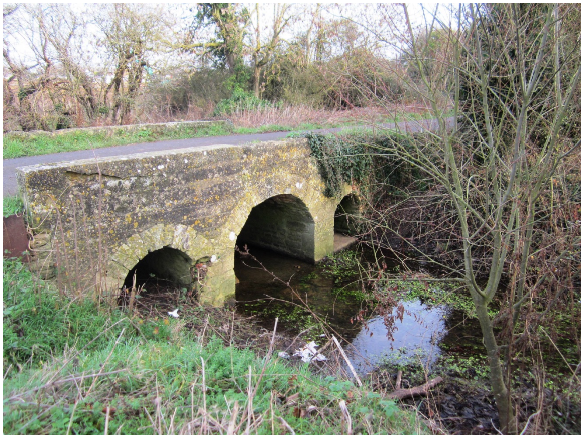
Plate 4: The grade II Chil Bridge (facing northeast with new development under construction in the background)
