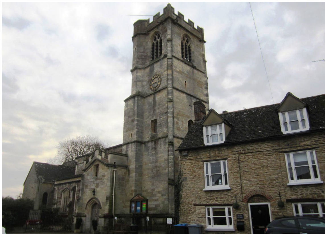
Plate 8: Grade II* Church of St Leonards (facing southeast)
