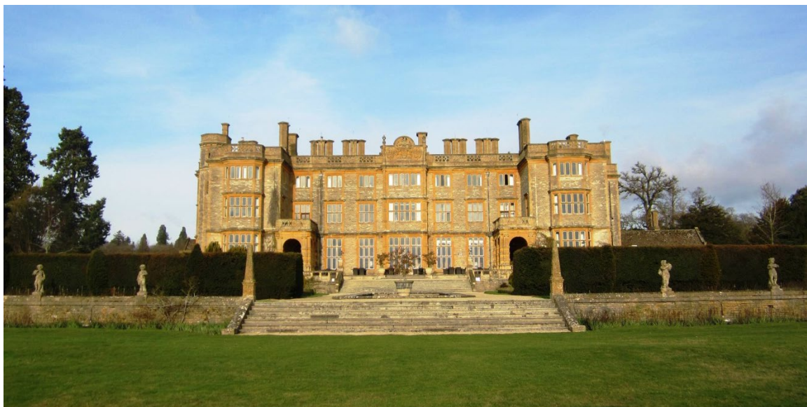
Plate 13: Eynsham Hall and terraces facing north
