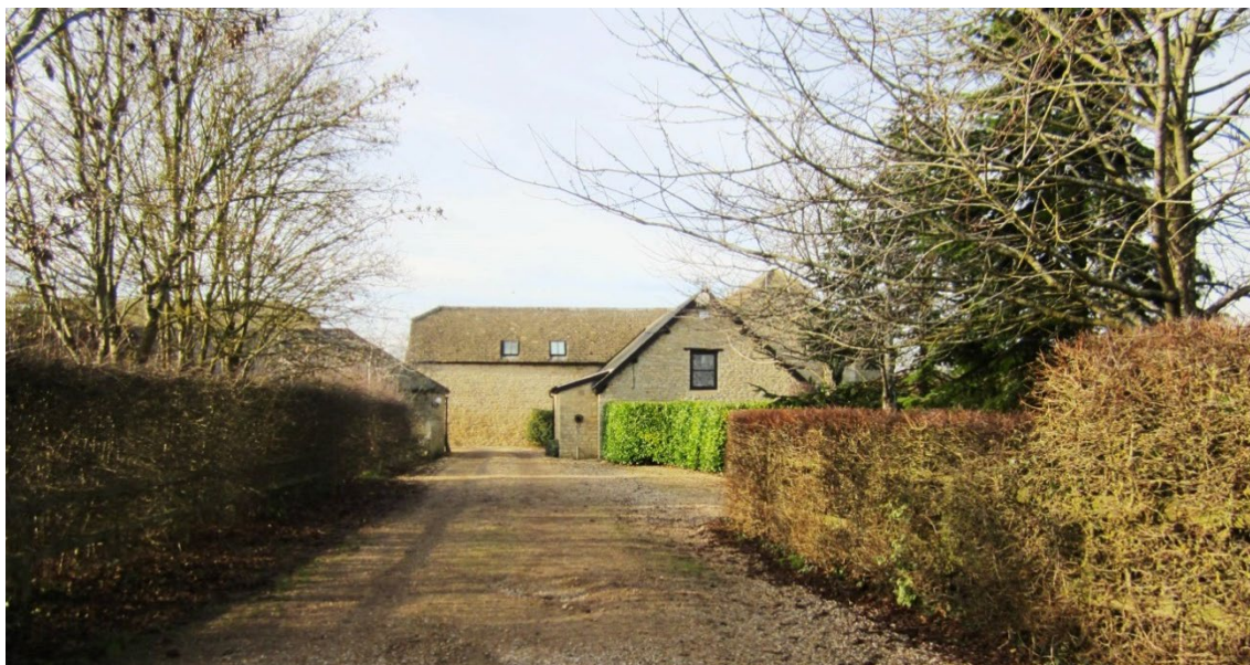
Plate 12: City Farm facing west
