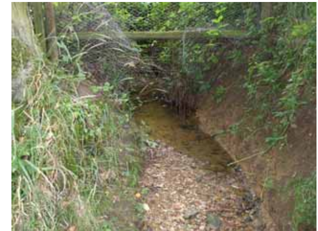
Area 4- Ditch at Stanton Harcourt Road
