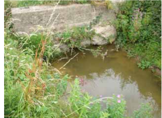
Area 1 – Culvert at Limb Brook
