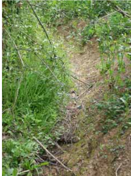
Area 1 – Badly defined ditch off South Leigh Road
