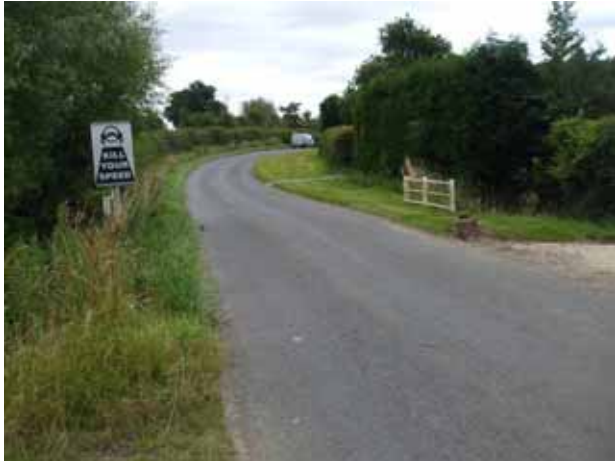
Area 1 – Culvert under South Leigh Road
