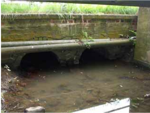
Area 3 – Brick arch culvert at Margery Cross
