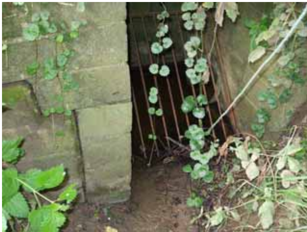
Area 4 - Culvert at Stanton Harcourt Road
