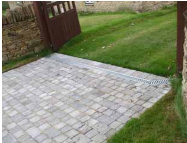
Area 2 – Cut-off drained installed at Chapel Road
