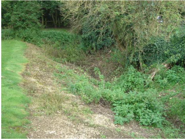
Area 3 – blocked ditch behind Lakeside flats
