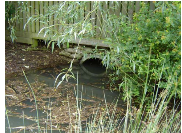
Area 3 – culvert at hotel boundary
