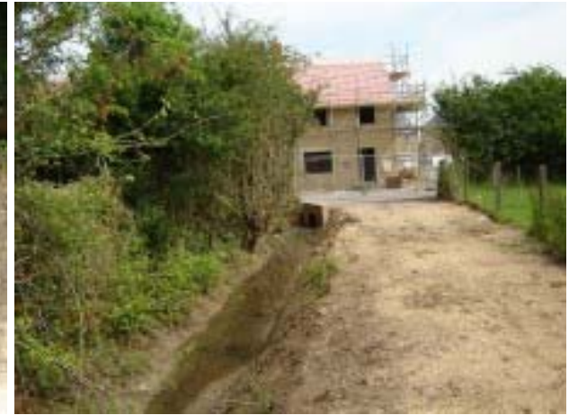
Area 1- Banner Homes Building site
