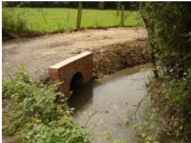
Area 1- Culvert crossing opposite building site
