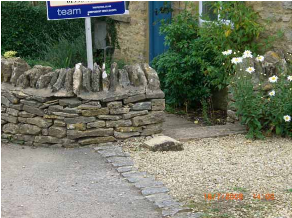
Threshold of affected property on Lower End below highway level, no kerbing to edge of highway.
