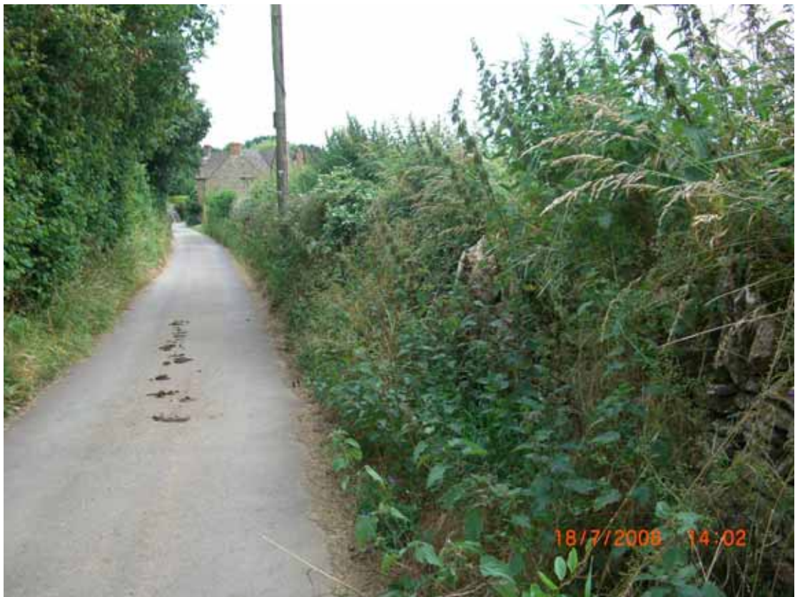
View south along Greenwich Lane towards affected properties. Again dry stone wall and grass verge prevent flood waters from exiting lane. Lane acts as a flood flow route, conveying water towards affected properties.
