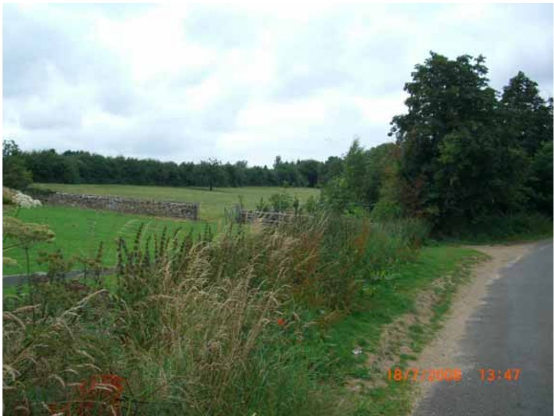
Surface water run-off from field affects properties on Buttermilk Lane. Mitigation proposals include re-profiling of field to direct flows away from properties.
