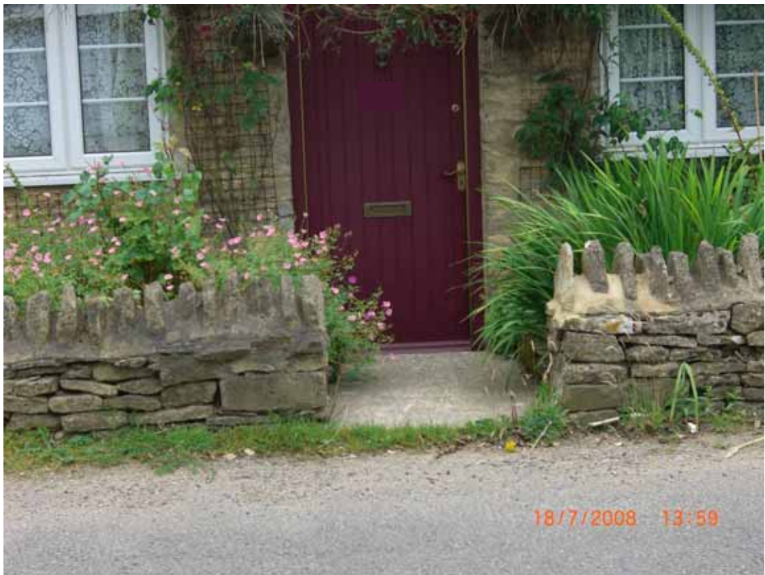
Threshold of affected property on Lower End below highway level, no kerbing to edge of highway.
