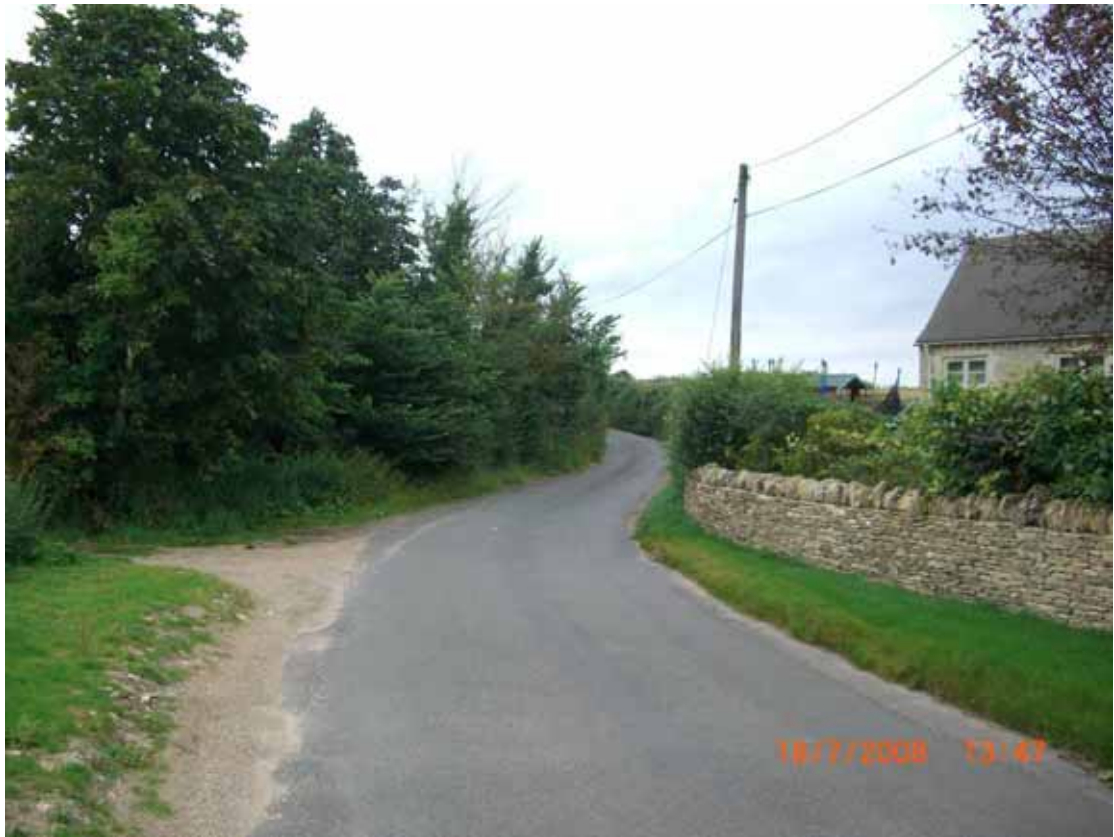
New boundary wall to property on Buttermilk Lane. Flooding affects two properties from fields and road to the north.
