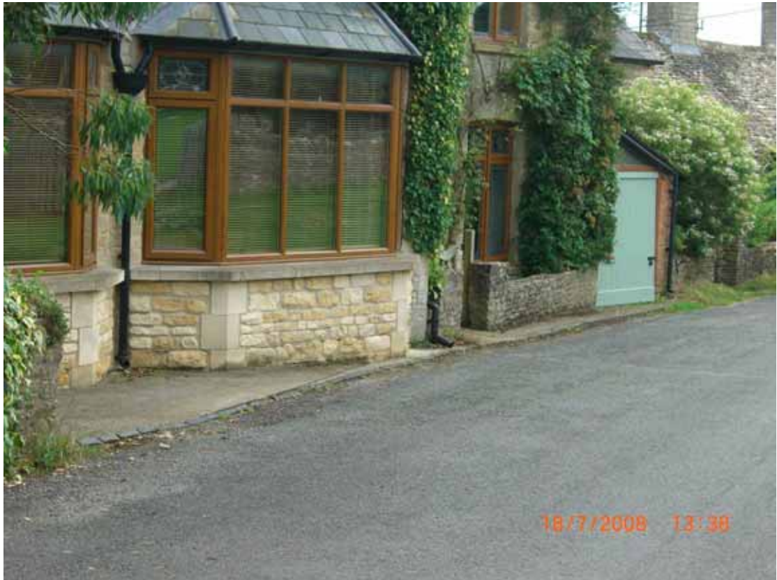
Low property threshold to the south of the village green. Also a visible lack of significant kerbing.
