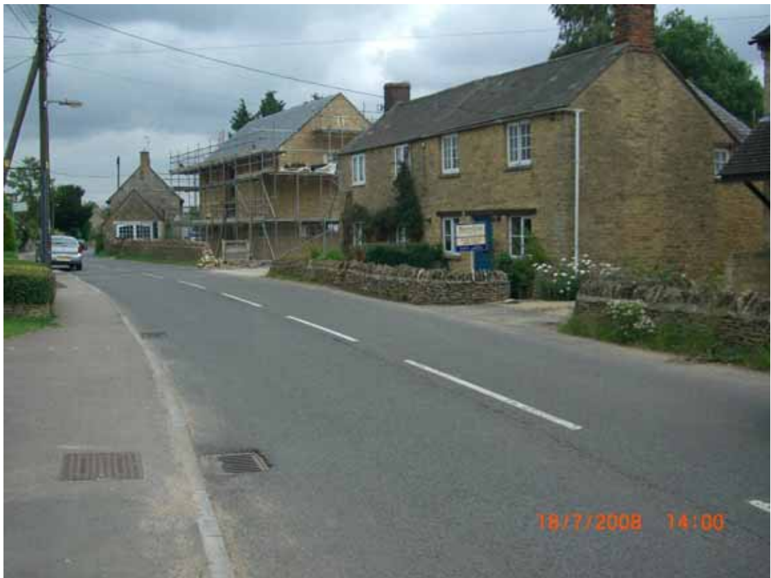
Gullies on northern edge of Lower End, no drainage shown adjacent to affected properties.
