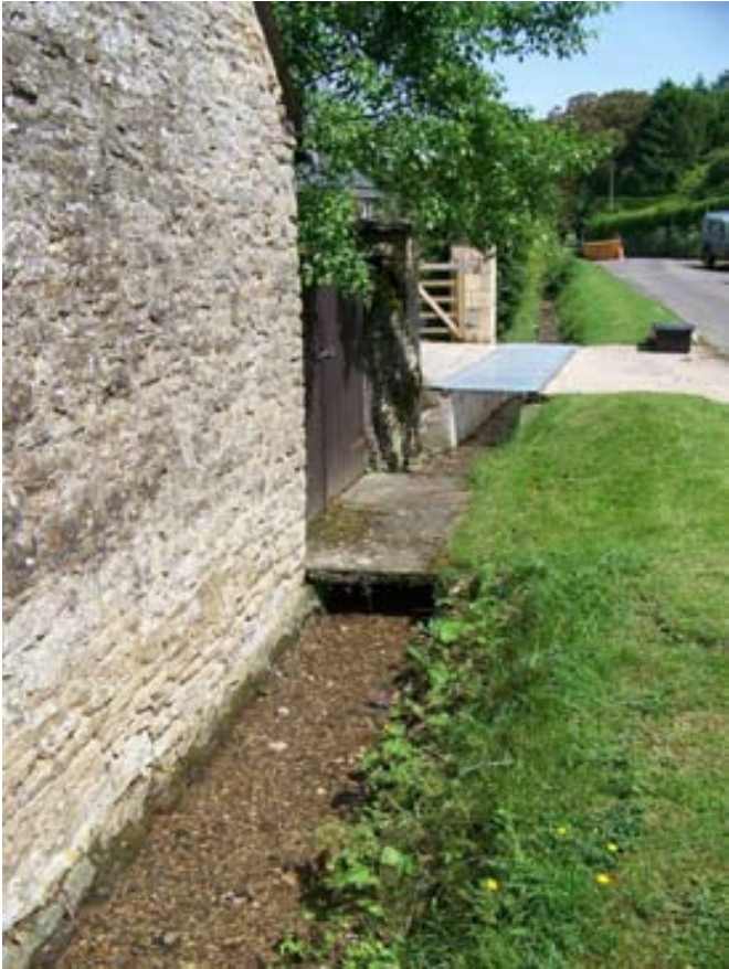
Photo 21: Clear, widened ditch outside properties
