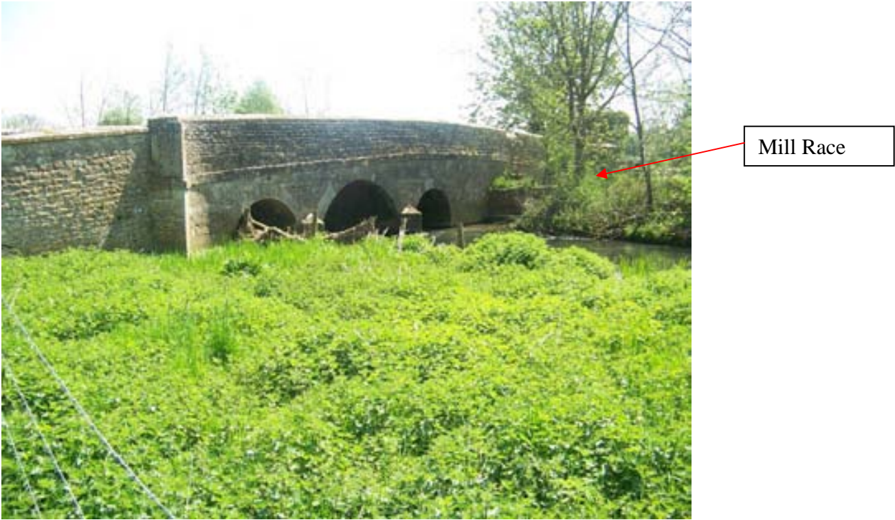
Photo 10: Bridge at Asthall over the Windrush and the Mill Race
