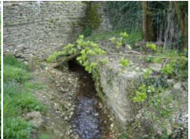
Culvert outlet watercourse at Ivy Nook, Kencot (area 1)
