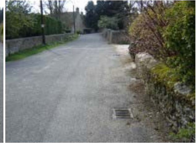
Highway drainage Kencot to Broadwell (area I)
