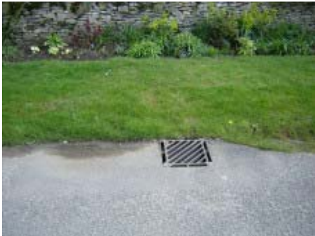
Highway drainage culvert vent in Kencot (area I)
