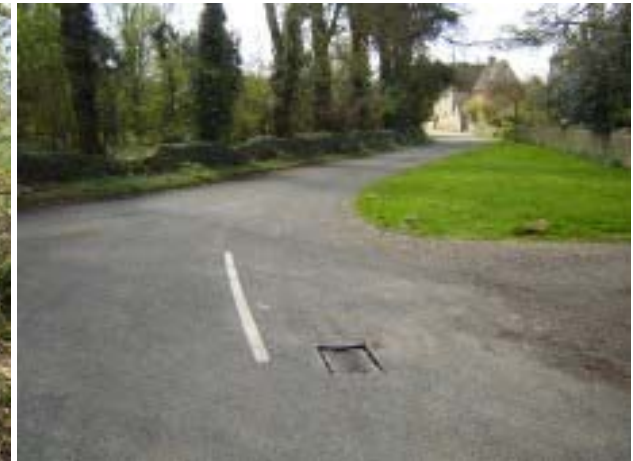
Highway drainage outside Kencot (area I)
