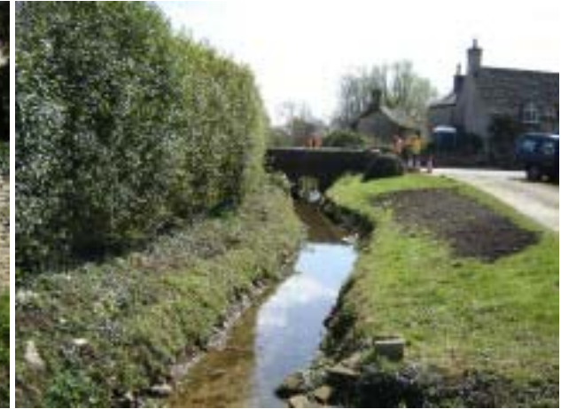
Kencot Bottom highway bridge (area 2)
