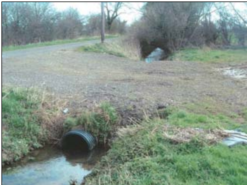
Photograph 14: Clanfield Brook running parallel to Calcroft Lane This photograph shows farm access restrictions to flow near to Bazeland Farm
