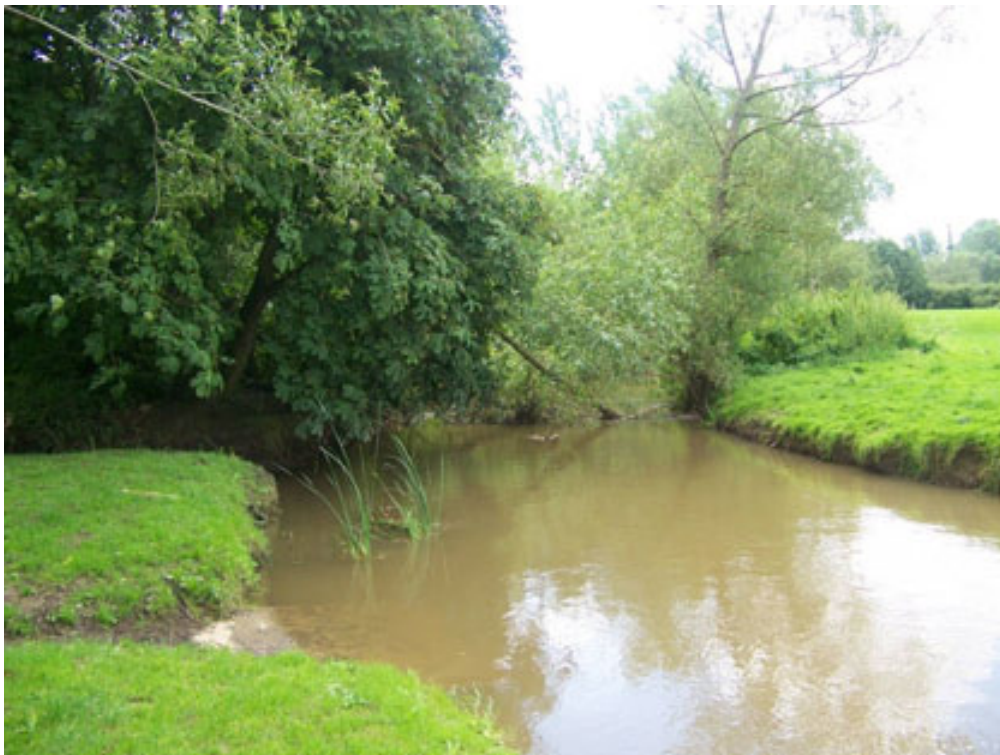
Looking downstream on the Mill Cut from Pound Hill / Water Lane (taken July 2008). Vegetation in the channel poses a restriction to the flow of water, although this situation has occurred since July 2007.
