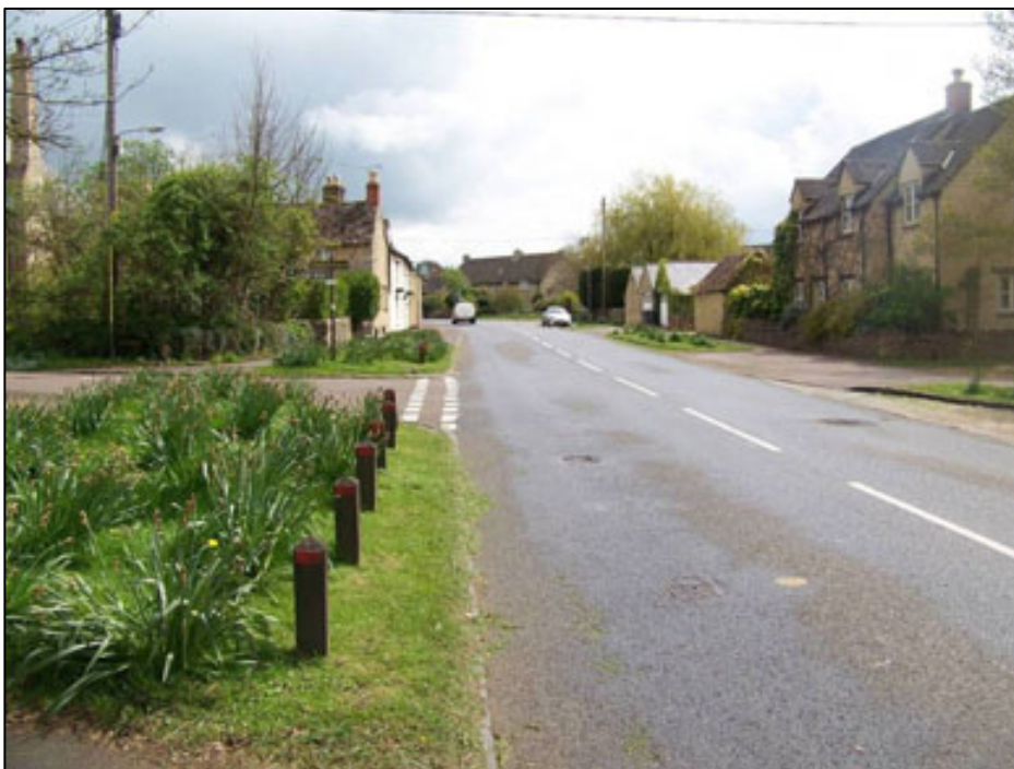
Photo 6: Station Road with Mill Lane on the left. This photo shows the low kerb line and level of property in relation to Station Road.
