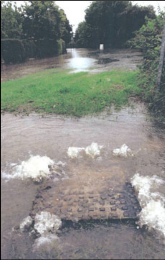
Photo 13 – Manhole surcharging at Lower End
