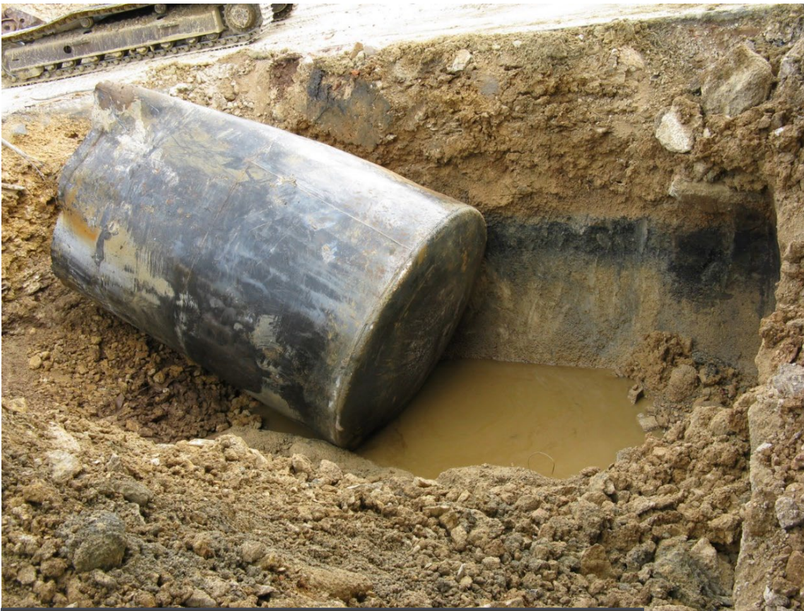
FIGURE 2 Disused tank with soil contaminated by leaked fuel, discovered at an industrial estate
