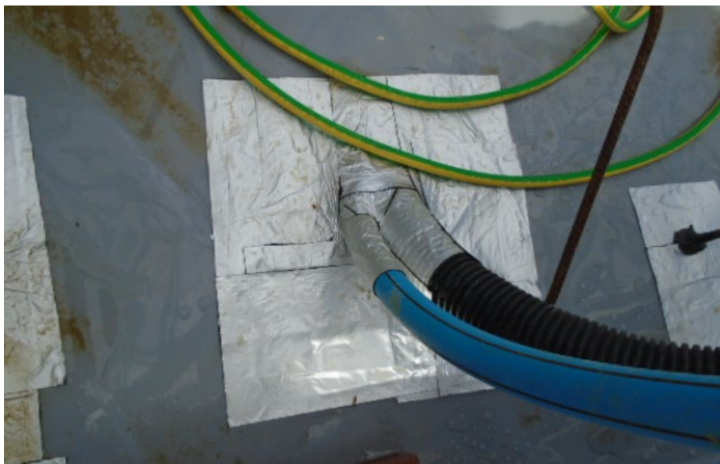
FIGURE 5 New floor slab with service penetrations sealed against ground gas ingress
