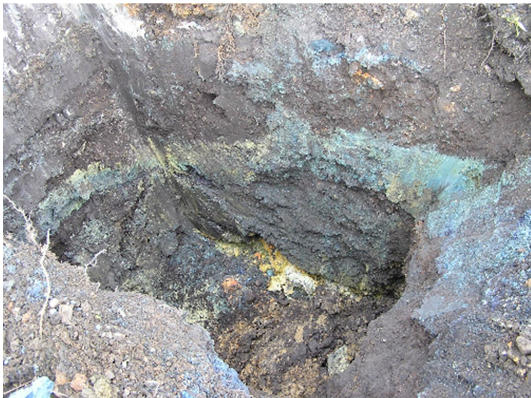
FIGURE 3 Contamination found under old slab base
