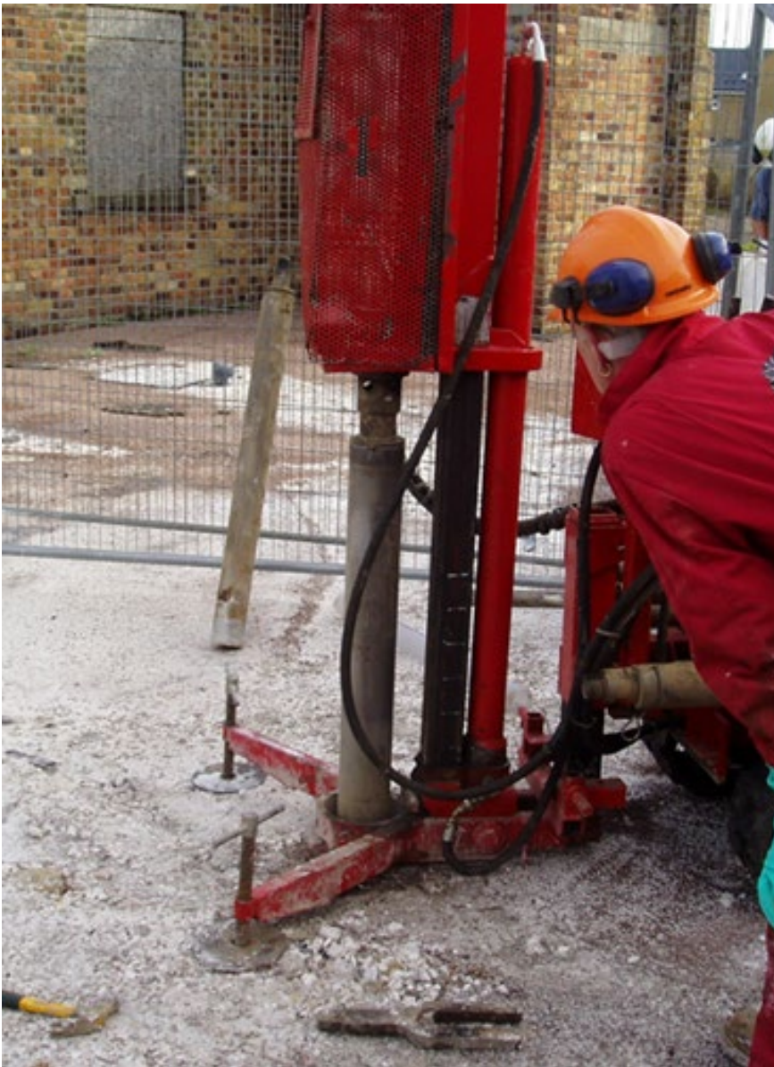
FIGURE 4 Site investigation in progress, borehole drilling for soil sampling
