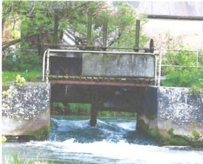
Source: Crawley Flood Prevention Group Report, Crawley Parish Council (April 2008)
