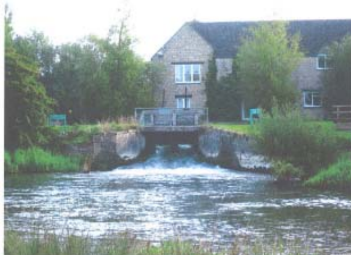
Source: Crawley Flood Prevention Group Report, Crawley Parish Council (April 2008)
