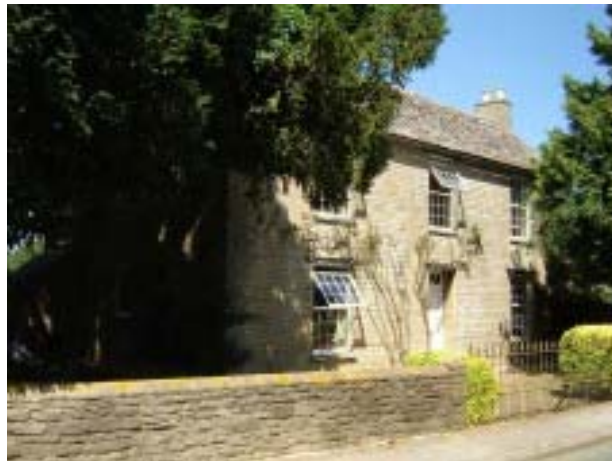
Area 4: Cote Villa, Cote Road
