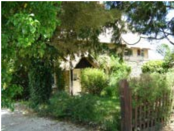
Area 1: Merton & Tanglyn Cottages opposite Aston Ditch tributary.
