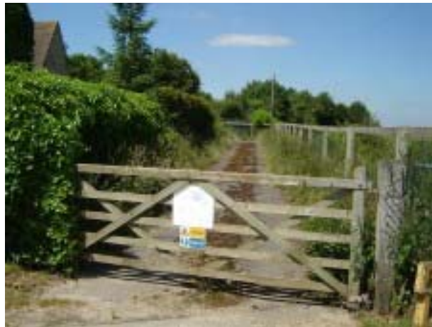
Area 2: Thames Water pumping station in Bull Street.
