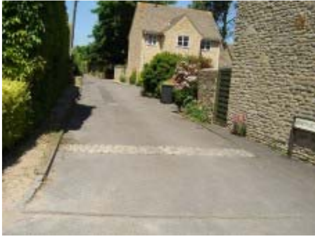
Area 2: Highway Drainage protection bund
