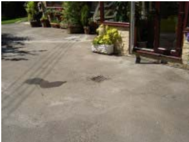
Area 4: Highway Drainage at Danelwood, Cote
