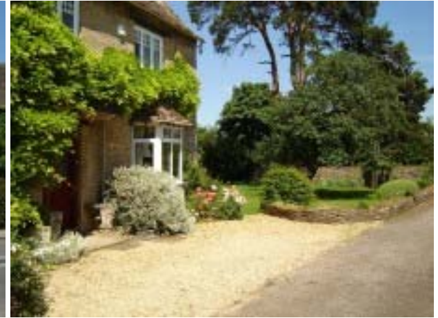
Area 4: Little End Cottage, Cote Road.
