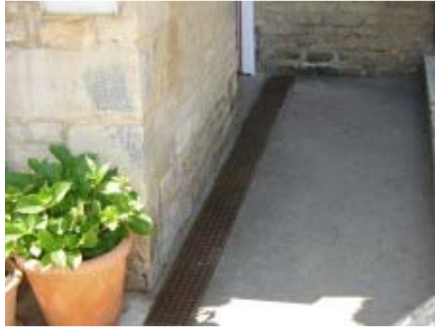
Area 2: Red Lion PH Threshold Drainage.
