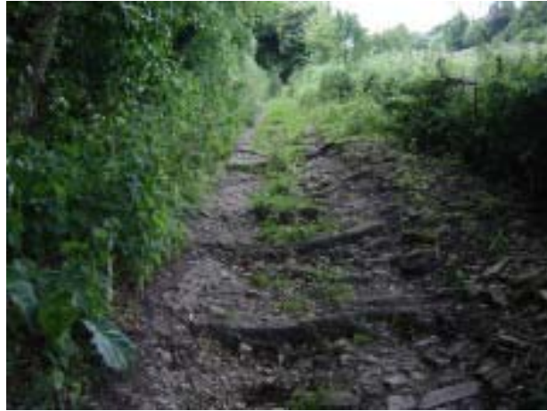
Area I - Water damage in Dark Lane
