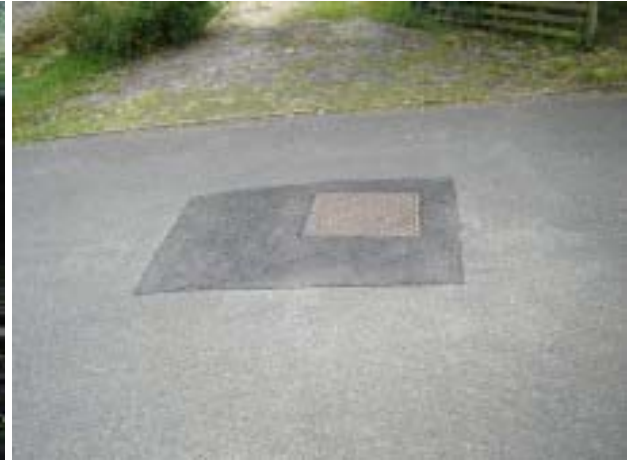
Area I - High Street repaired manhole damaged from surcharging
