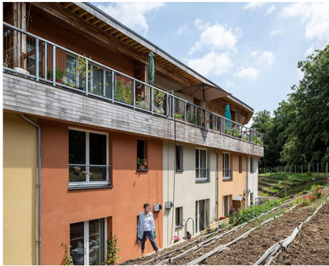
Image source: Anne Thorne Architects
