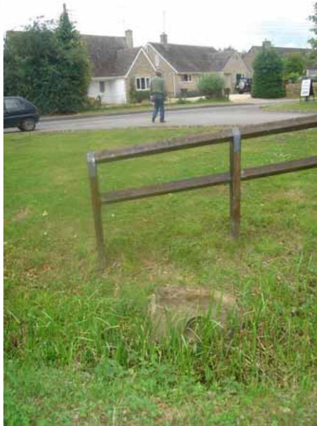
Area 2 – culvert from highway gully outfalling into hotel ditch
